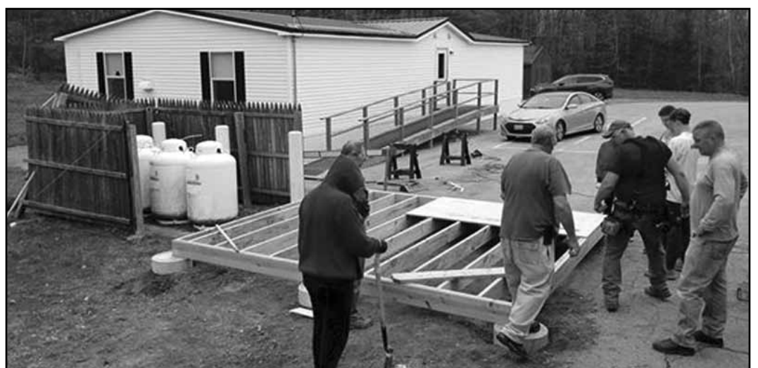
Volunteers install the decking.
